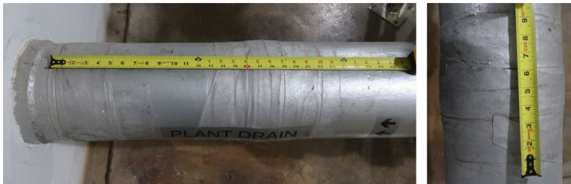
Figure 17.—Fiberglass wrap repair on 8-inch diameter unwatering piping.
